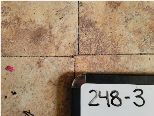
248-3 12"x12" Floor Tile/Mastic Interior Living Room (Bottom Layer)
