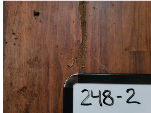
248-2 Laminate Flooring Interior Living Room (Top Layer)
