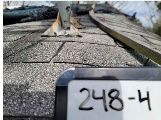
248-4 Asphalt Shingle Typical Exterior Roof
